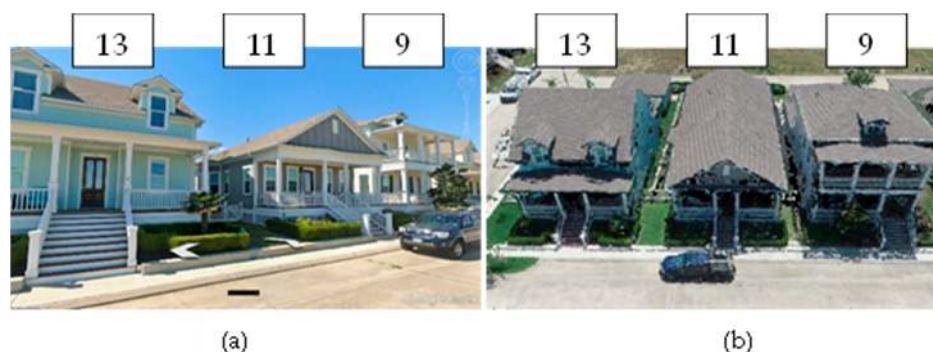
Figure 4. Housing addresses Sunrise Row 13, 11, and 9 located in the Evia community seen in (a) google street view (GSV) and (b) screenshot of Pix4D DPC.
