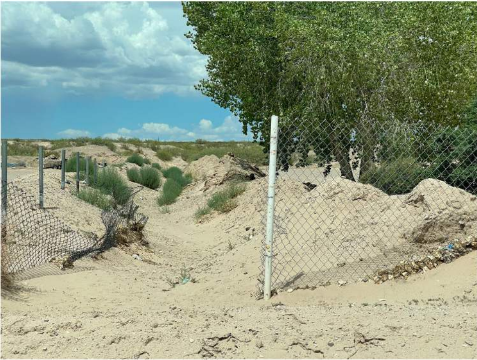
Figure 1. Photo of an arroyo (dry creek bed) that becomes a rushing river with as little as half an inch of rain.
